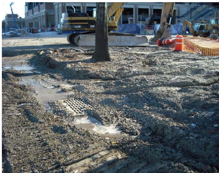
No protection fencing – concrete washout without silt fencing. Credit: N. Zürcher
