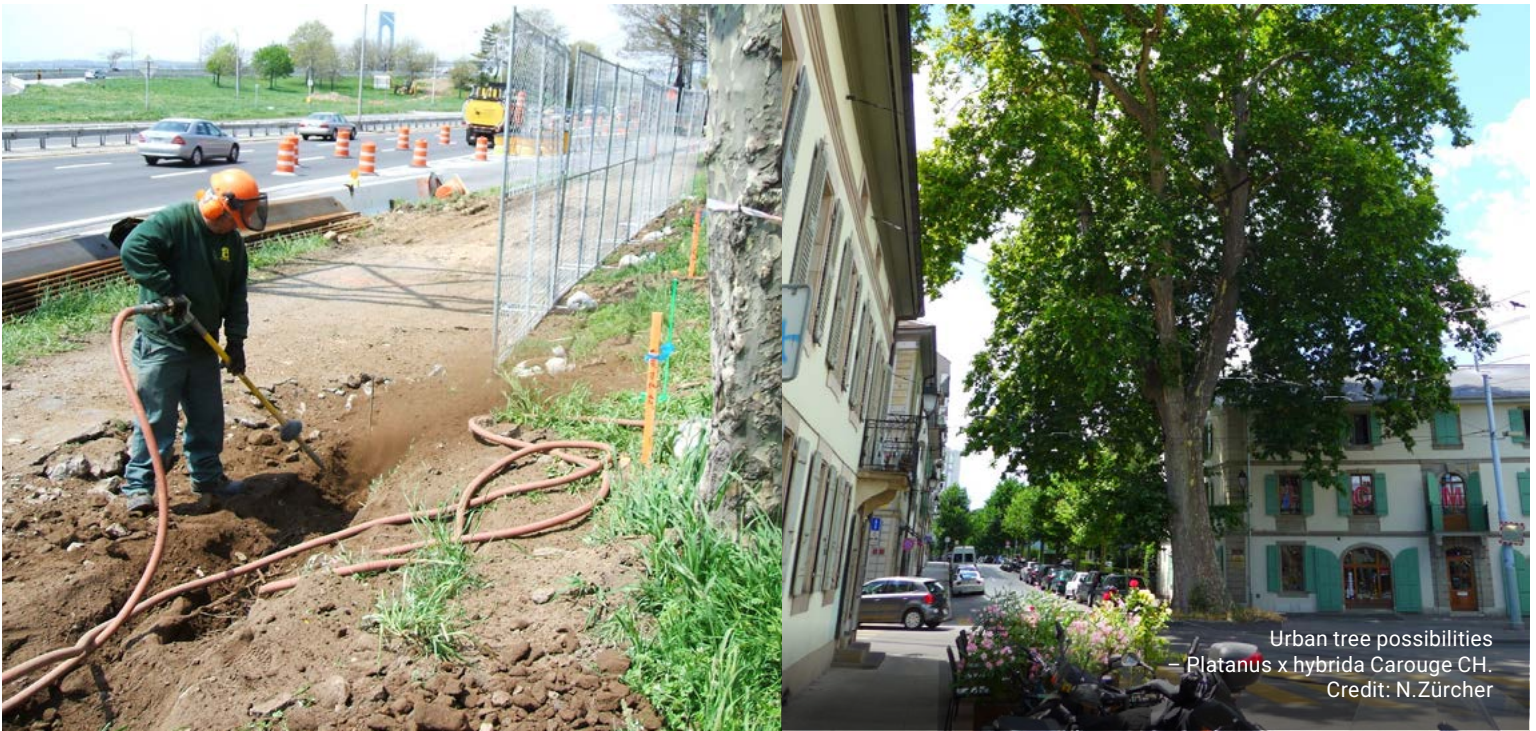
AirSpade® excavation for root pruning. Credit: N. Zürcher
